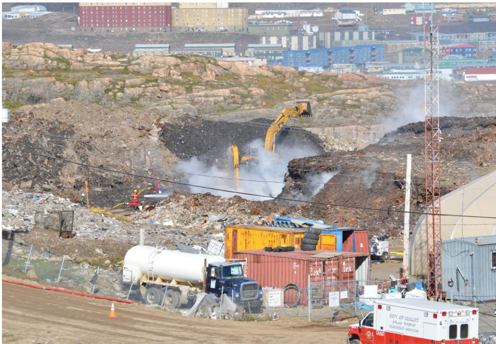
The Iqaluit 'Dumpcano' smouldered for several months during the summer of 2014. Credit: Aaron Watson
